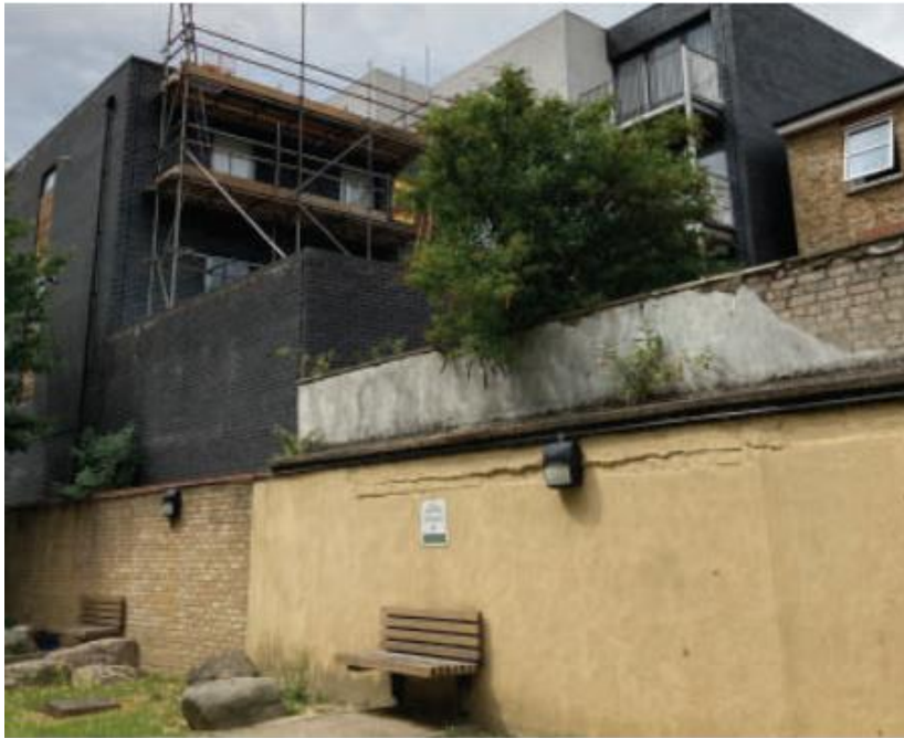
Rear elevation as viewed from garden associated with Cadel House
