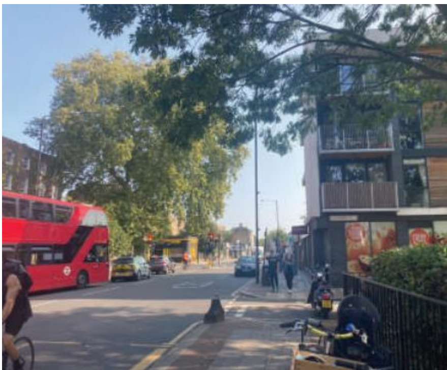
West elevation as viewed from Hackney Road
