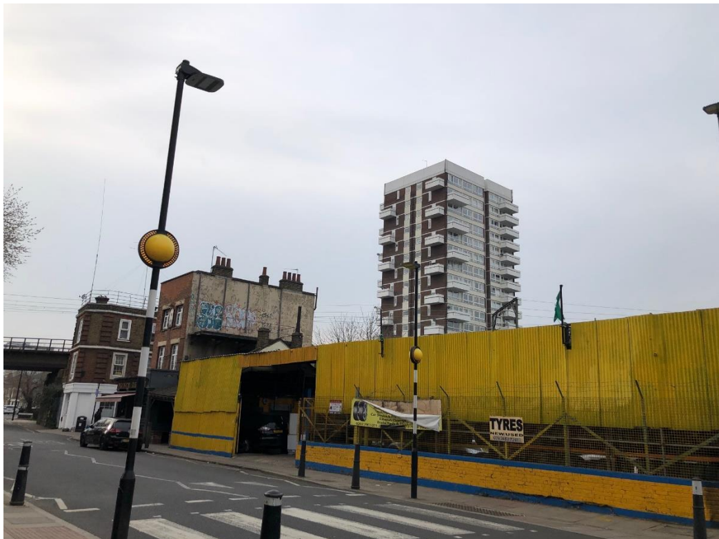
View from Salmon Lane looking West, with the flank wall of the Prince Regent Pub siding the site.
